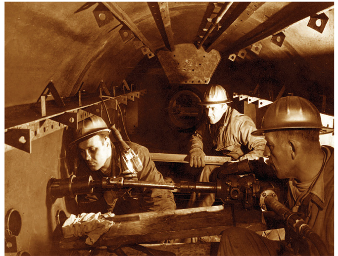
Rolling tubes, Boilermakers at work
